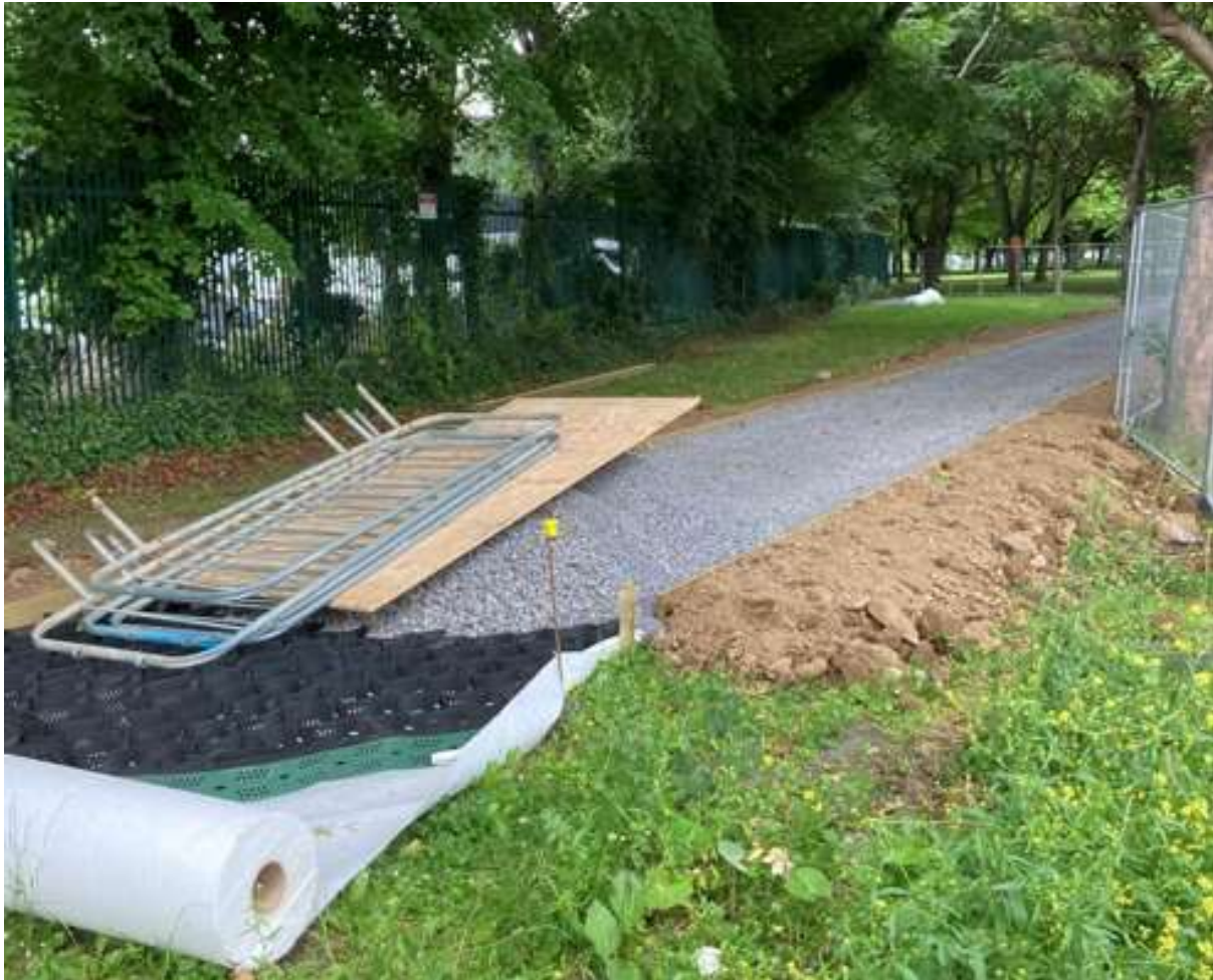
Figure 3-79: Tree root protection system under new tarmac path in Fairview Park, Dublin 3
